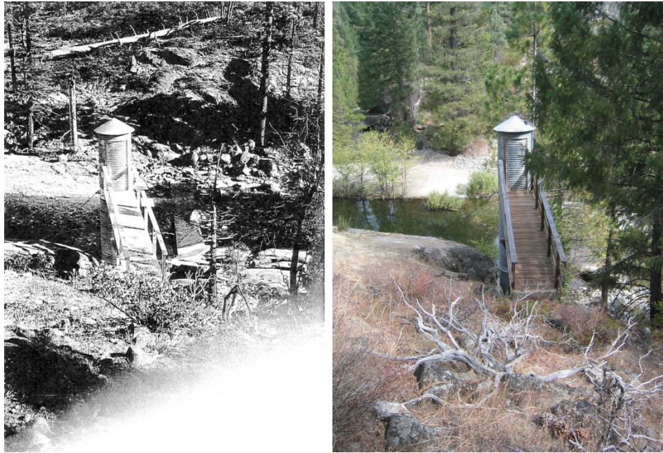
Figure 6-14: Upper Cherry Creek at the USGS Gaging Station Control (Cherry Creek below Cherry Valley Dam) in 1953, Compared with 2006 at Same Location. Note Extensive Riparian and Upland Encroachment into the Channel, and Cobble/Gravel Spoils on Opposite Bank from USGS Maintenance of Deposited Coarse Sediment.
